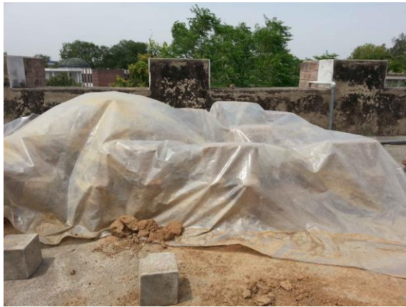
b) Bricks Covered with Plastic Sheet
