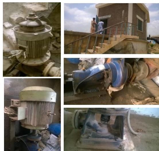
Fig. 3: Condition assessment survey of TW, OHR, GST
