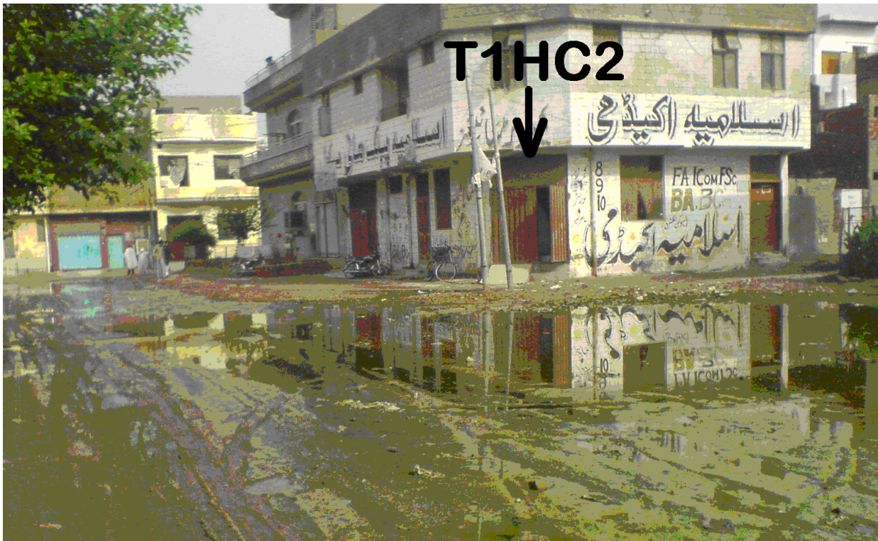
Fig. 7 Stagnation of sewage in front of house connection T1HC2
