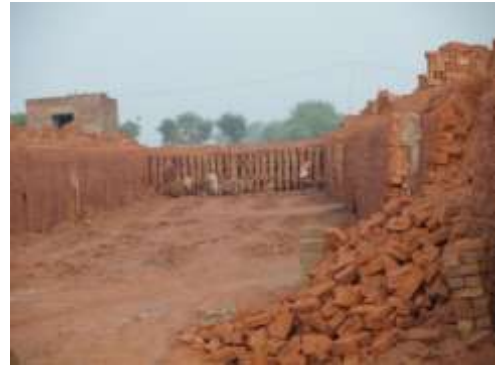
Figure 8: Brick specimens removed from kiln
