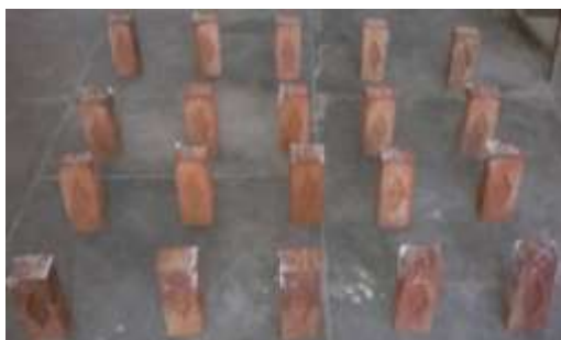
Figure 15: Efflorescence observed on brick specimens after 45 days
